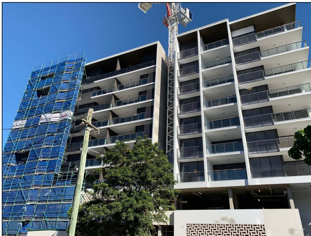
Eastern façade from street level
