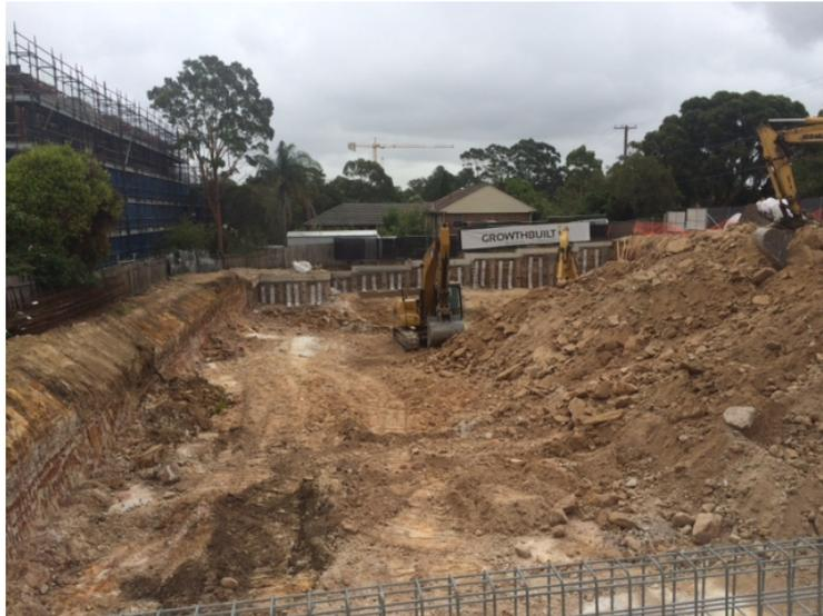
Photo 2: Below is a photo showing the drainage cell and reinforcement completed ready for the concrete placement. The bulk earthworks has also commenced to the second basement
