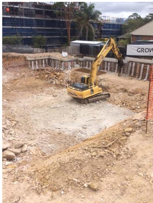
Photo 3: This photo was taken on the 10/12/14. As you can see the concrete to the first drop of shotcrete has been completed on the western side. The reinforcement and drainage cell has also been completed for the second drop awaiting the concrete to be applied. The reinforcement has also been installed over the sewer diversion works on the southern side.
