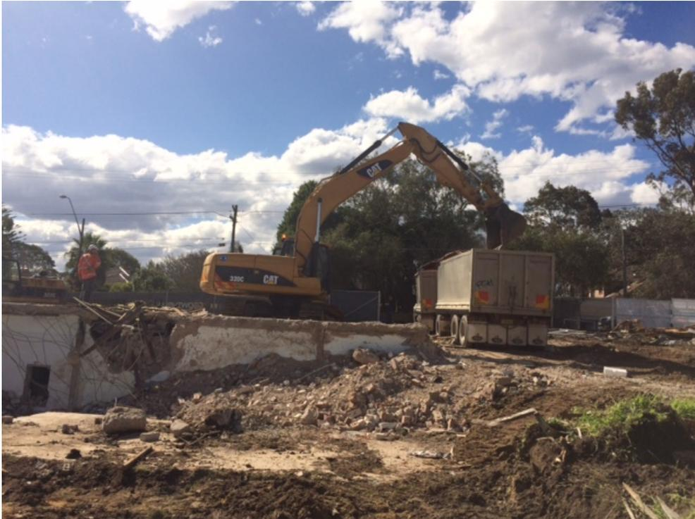
Photo 4: Demolition to No.606 has commenced as seen below. In this photo you can see the second excavator demolishing this building while the other is loading out the demolition material
