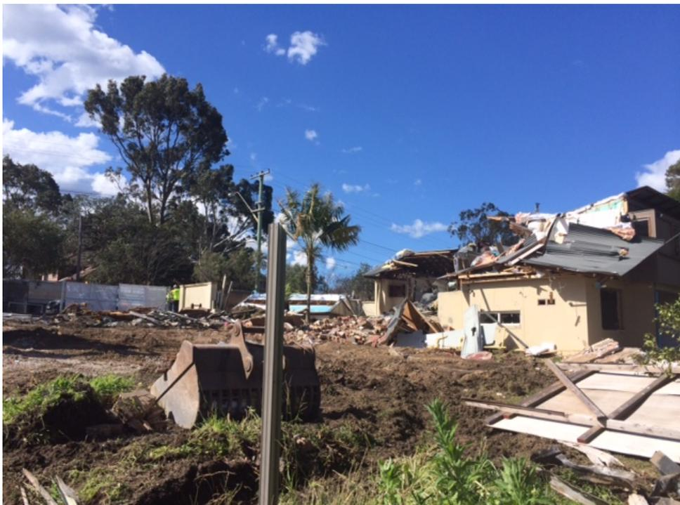
Photo 3: Demolition to No.604 has almost been completed in this photo. The 30 Tonne excavator is loading out some of the last demolition material of this dwelling
