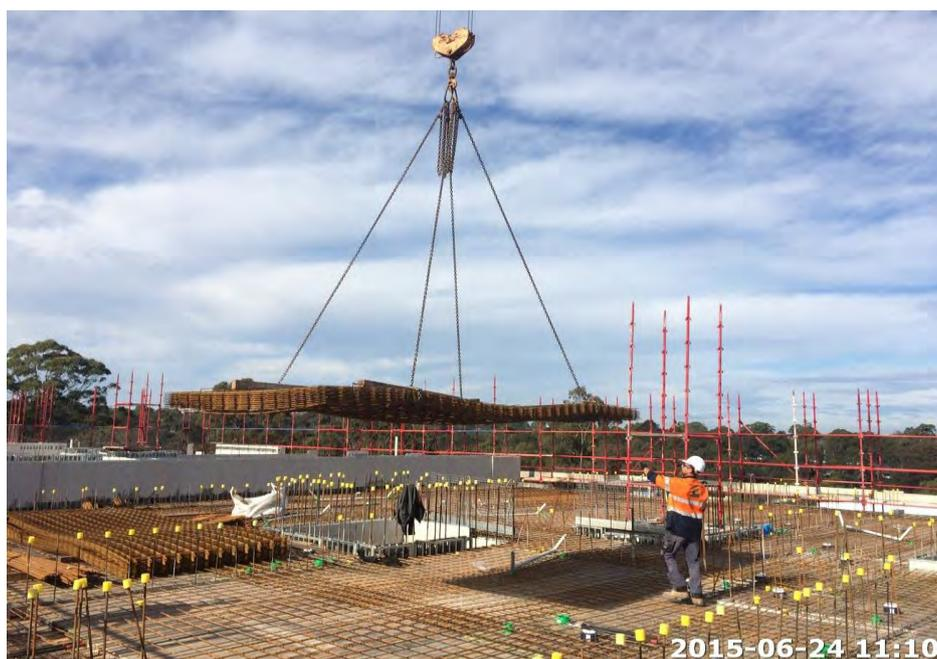
**Photo 3:** Shows the installation of the AFS walling system and bracing details on Level 2 East Deck. Once the formwork and internal AFS walls are completed the Level 3 deck sitting above can be prepared. The Level 3 concrete pour is scheduled to occur in the first week of July 2015. In addition to the AFS bracing, you can see the set-down area for the proposed bathroom area, and stacking of formwork. Note: The internal AFS wall cavity still requires internal reinforcement and concrete.
