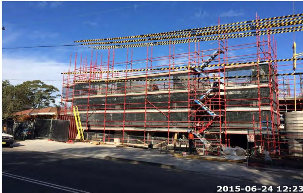
**Photo 2:** Shows the delivery of steel reinforcement (mesh) to Level 3 West Deck. All formwork and edging for the deck is completed, majority of steel reinforcement has been fixed, the AFS internal and lift shaft walls have been poured with concrete, hydraulic and electrical services installed, with the concrete pour scheduled to commence on 26/06/15.
