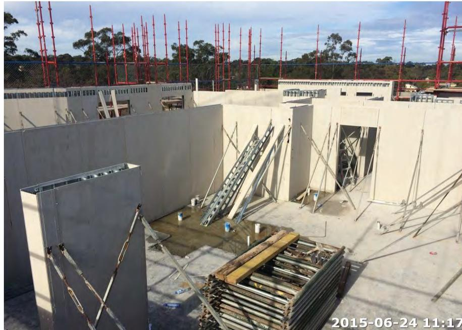
**Photo 4:** Shows that stripping of formwork and cleaning on Ground Floor West has commenced. This will free up the Ground Floor units to start receiving the finishing trades including internal studwork, sheeting and services rough-ins.
