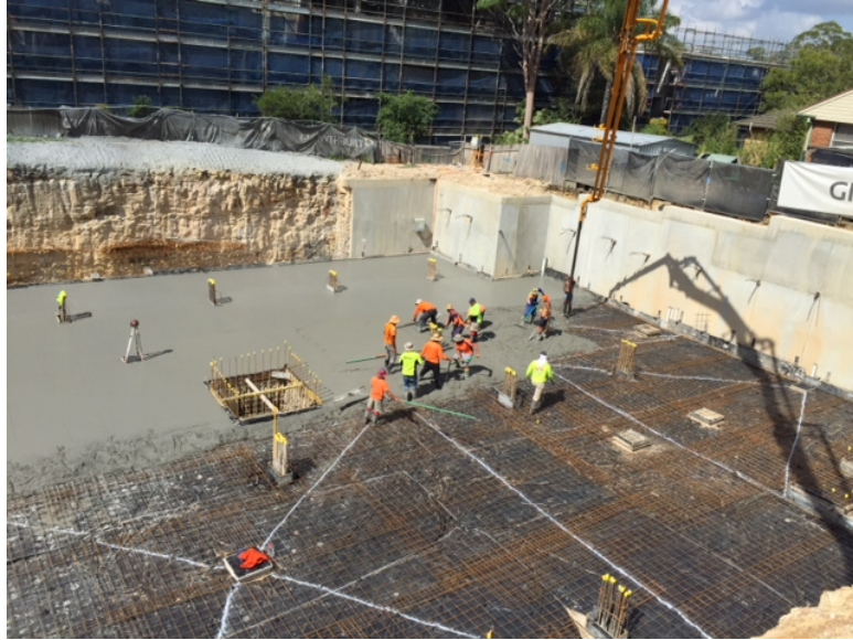
Photo 1: Basement 2 western side basement pour.
