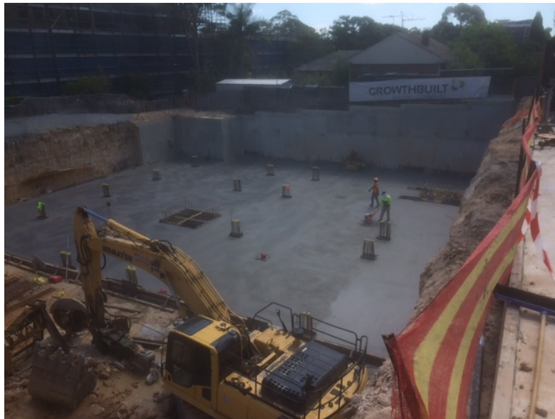
Photo 3: The completed slab
