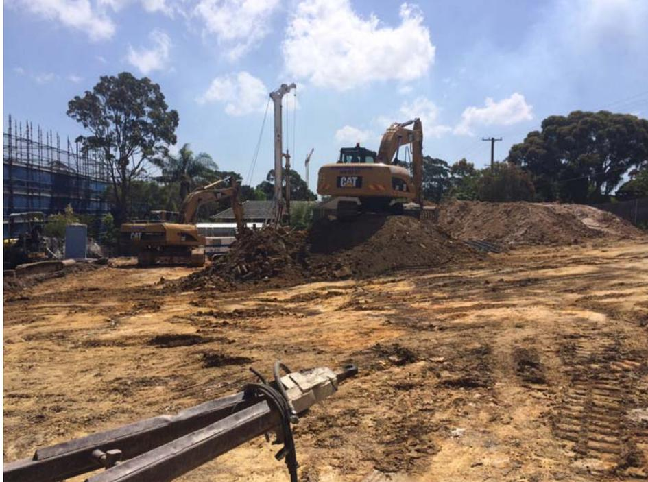
Photo 4: This photo shows the piles which have been drilled by the drilling rig. The reinforcement and concrete has been placed in the holes. These are the holes around the sewer diversion works
