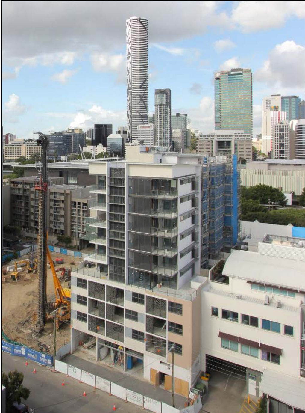
Figure 1: With scaffolding removed, the building façade is revealed.
