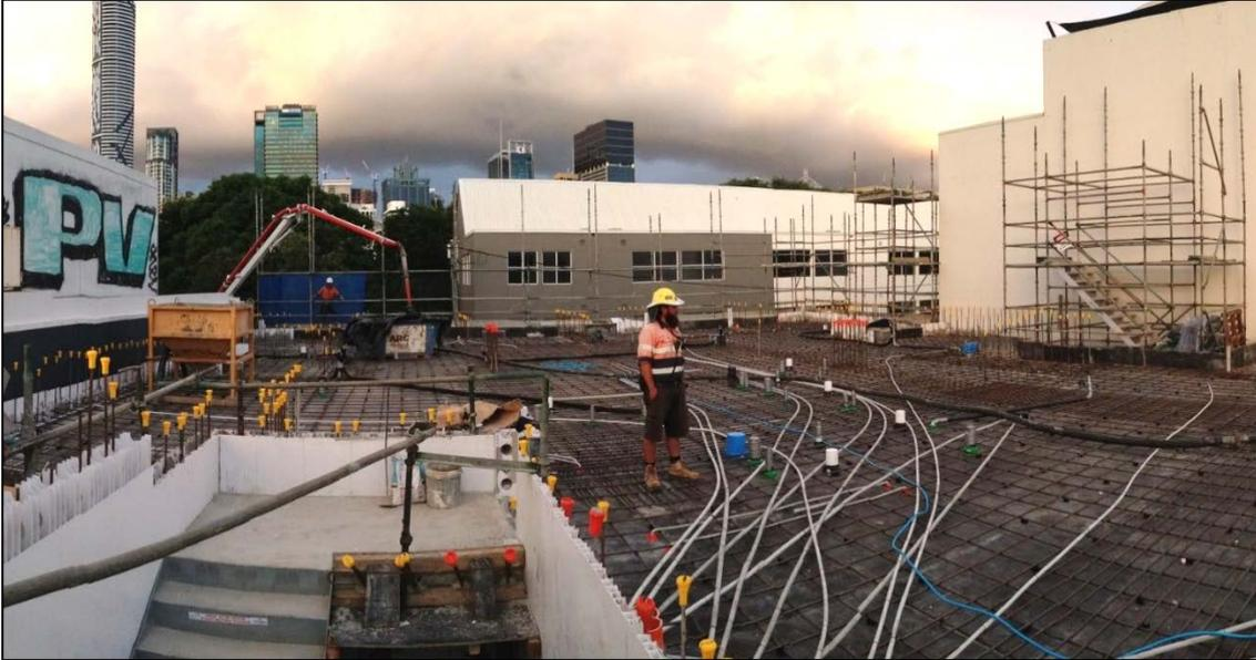
Figure 1: Site as viewed from Level 3 towards the city. Scaffolding and formwork in place for the level 3 slab pour.
