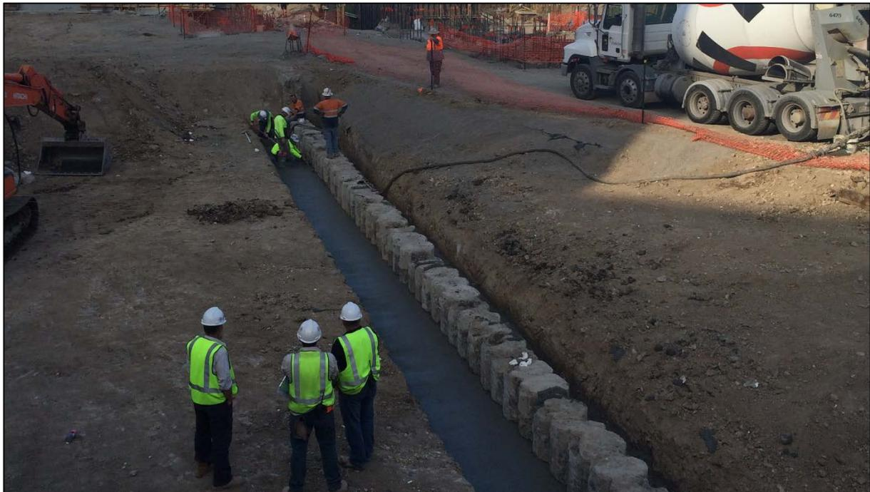
Haven Site: Secant retaining wall with the piling cap having just been poured. The tops will be trimmed off when the fresh concrete has cured.
