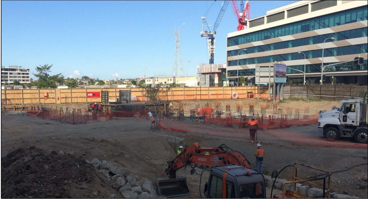
Haven Site: Foundation piles for the basement. The piles reach approximately 35m down to the bedrock.
