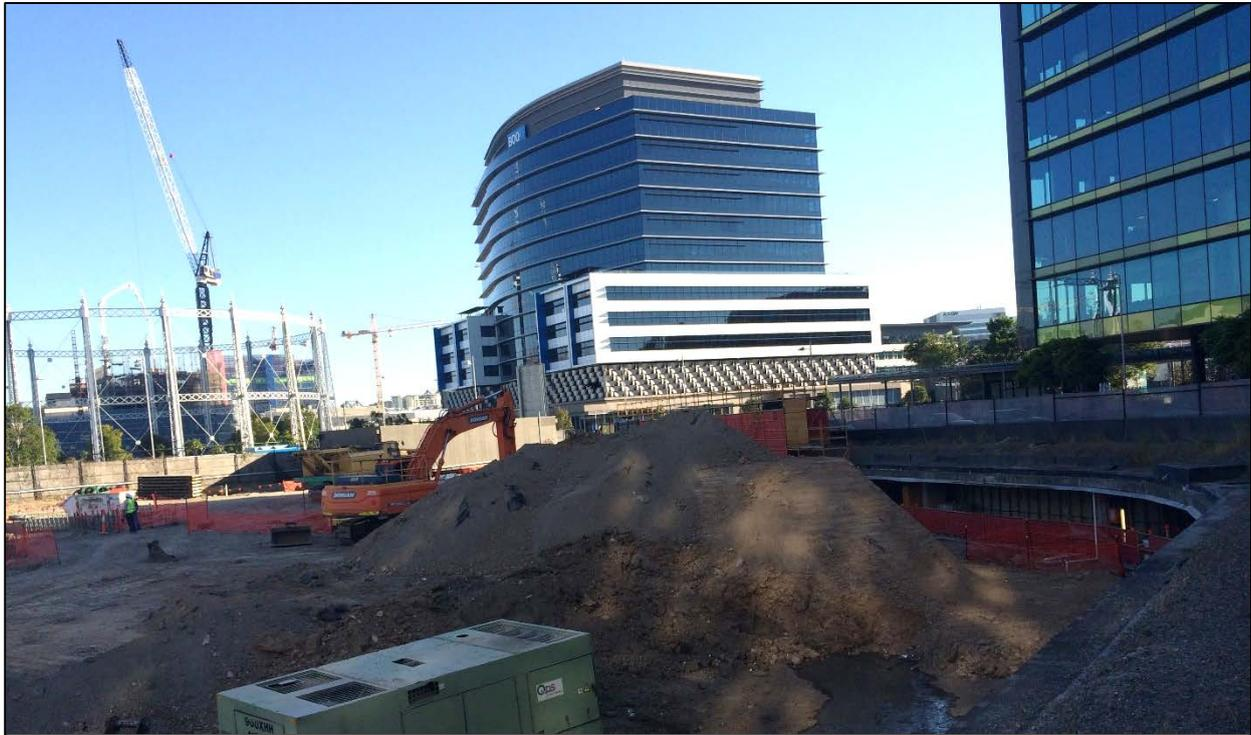
Haven Site: Pile of imported fill used to establish platforms for piling rigs. The material is now in the process of being removed from site.
