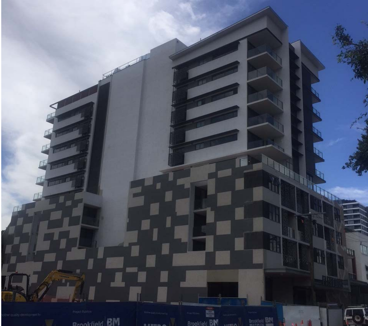
Figure 3: View from Hope Street - west side of the building.
