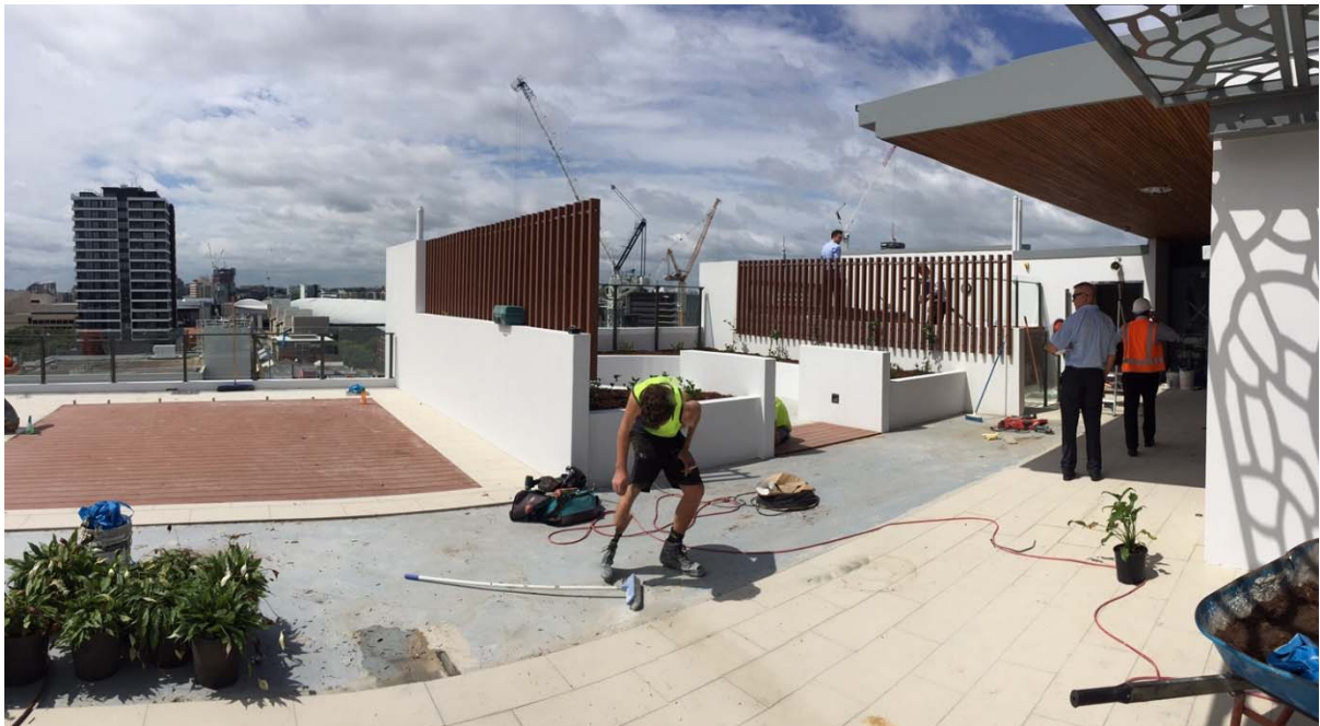
Figure 6: Roof-top terrace with Yoga Garden being installed.
