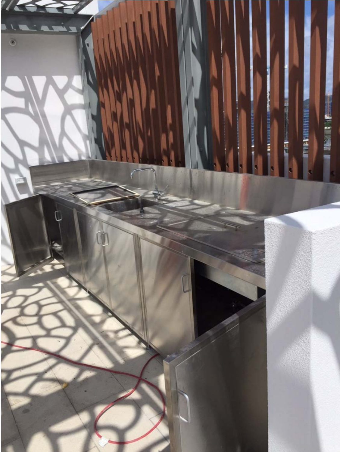
Figure 7: Roof-top terrace - BBQ being installed.
