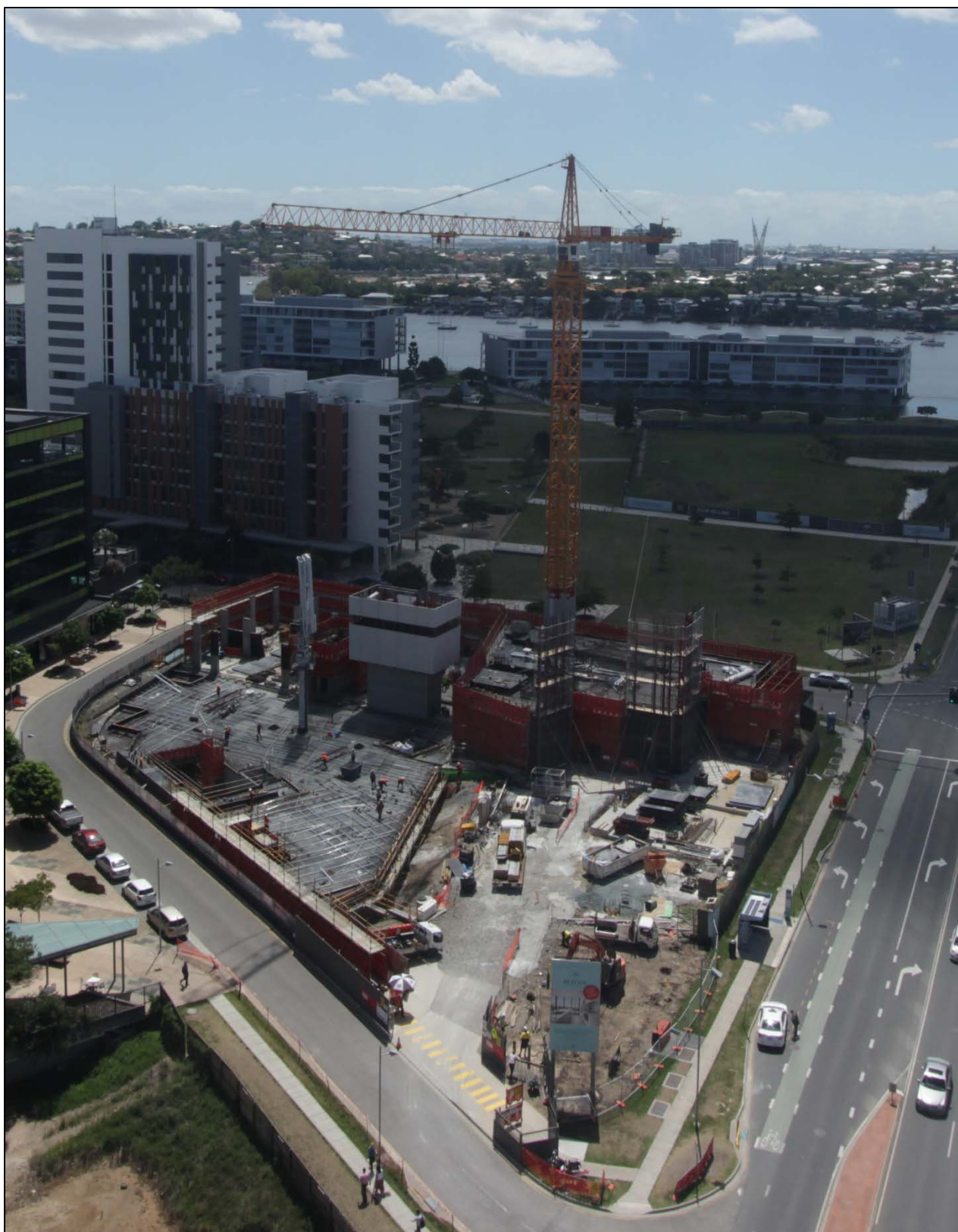
Haven Site: Construction Progress 15 th February 2016
