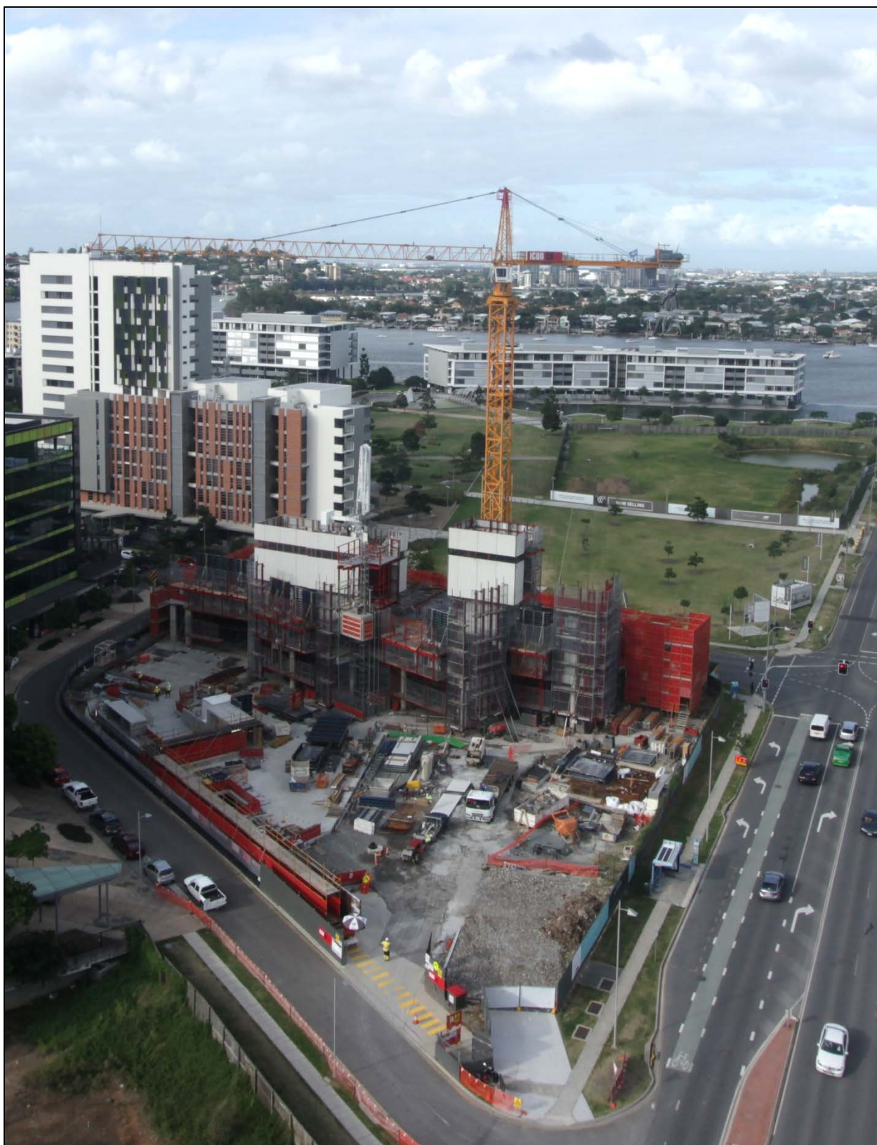
Haven Site: Site Photo 14 th April 2016
