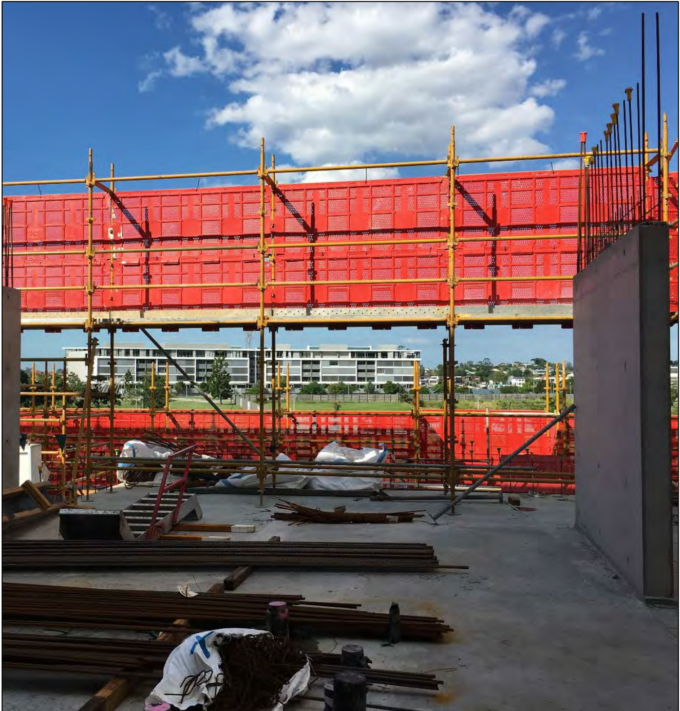
Haven Site: Park view from Level 1 apartments. Concrete blade walls will continue the full height of the building.
