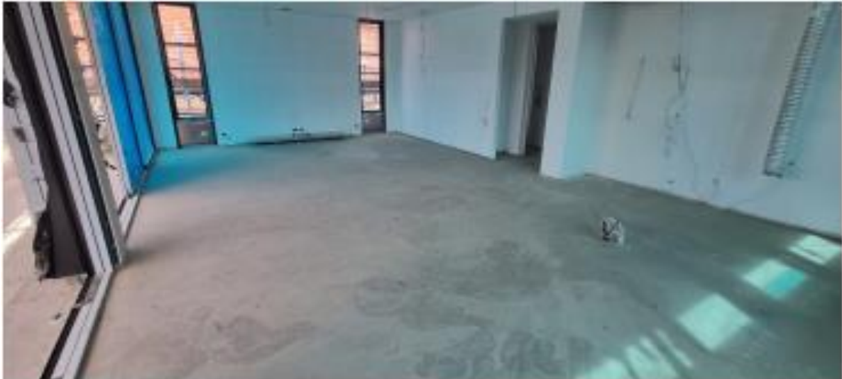
Floor Preparation & Topping completed on Level 2
