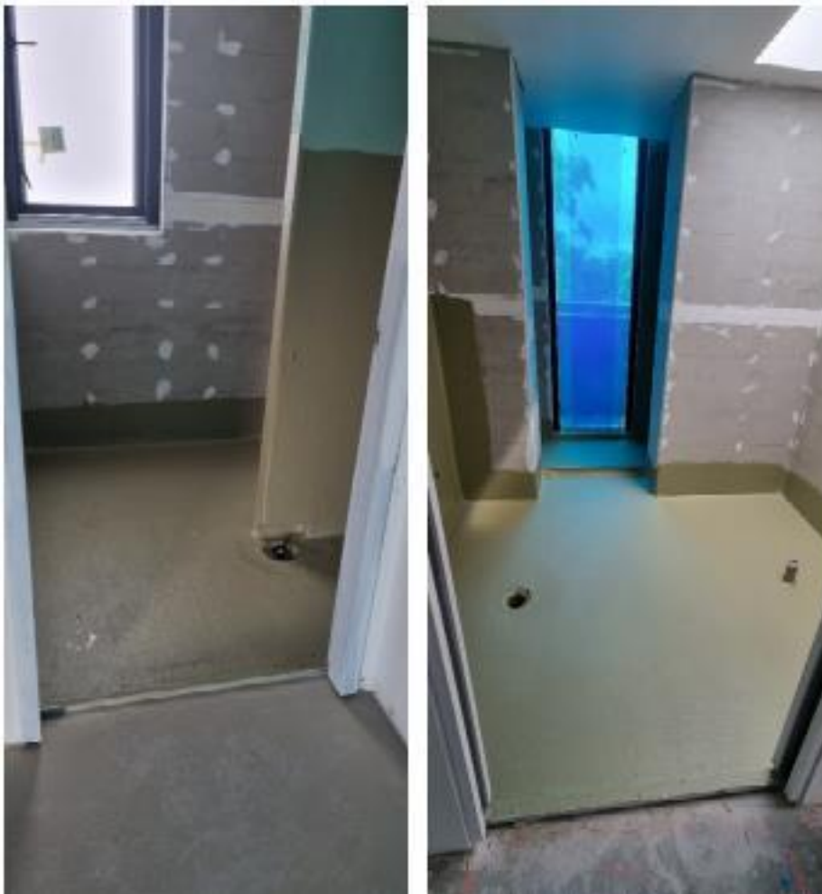
Waterproofing on Level 2 – 302 Ensuite
