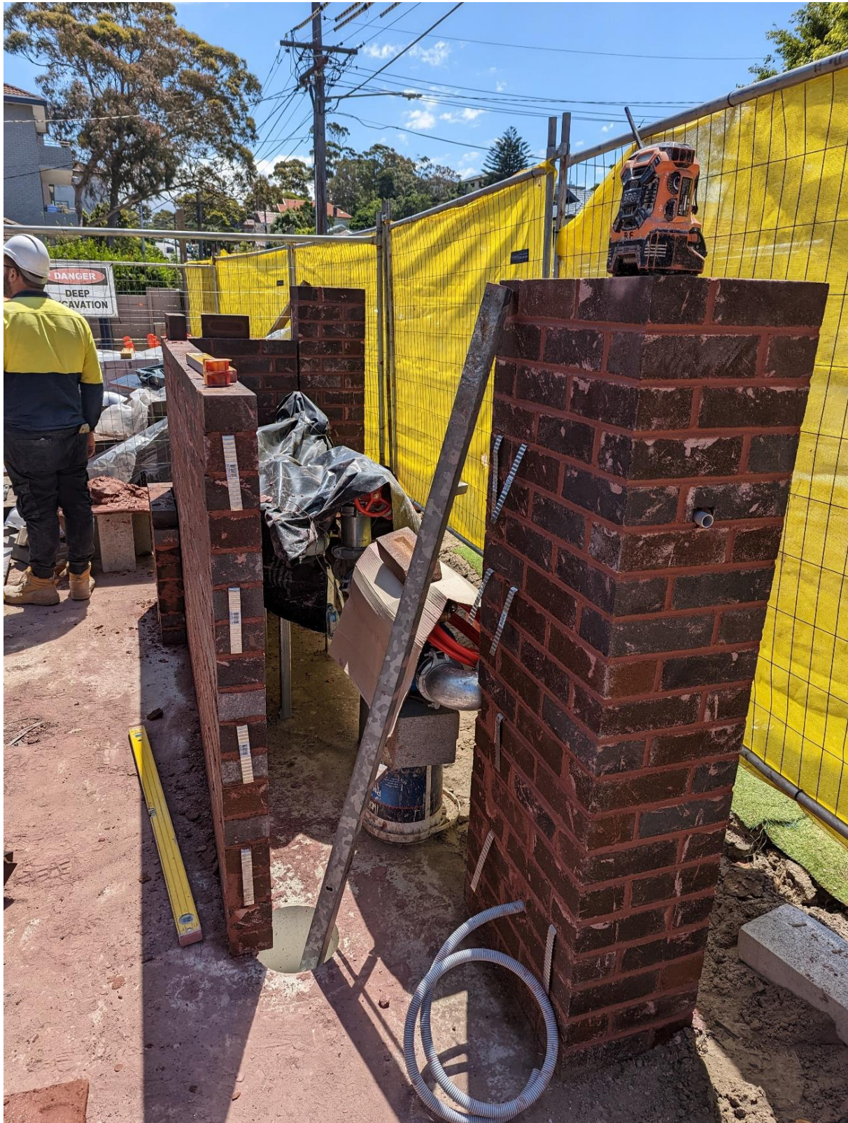
Frontage brickwork and booster cupboard
